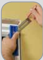
Lay Out Mitered Corners
